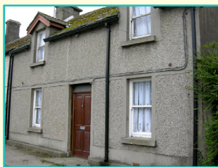
Kearney House Site
